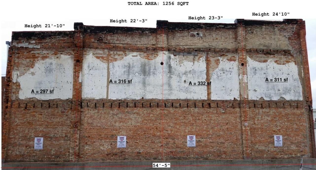
The building side will be prepped with an EFIS (Stucco) finish which will provide a solid color and surface for the mural. The base color can be white, other color options are available.
